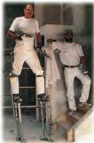
Son, Mark, and Jay dry walling a house
